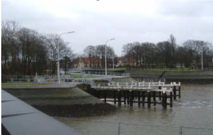
Sluices at Nieuport today.
